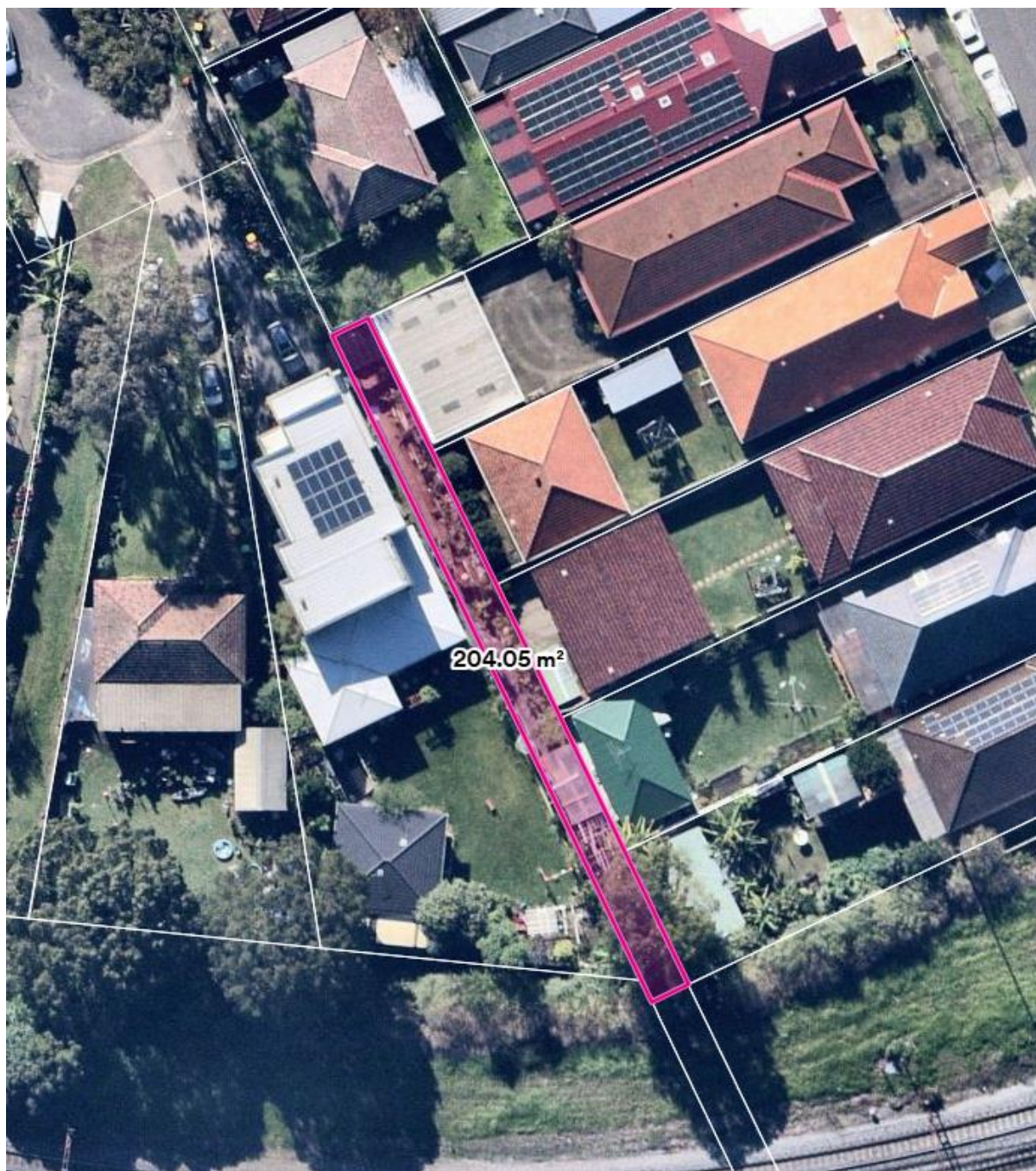
Figure 7. Aerial photo of Site 6, 1A Lincoln Street, Campsie
